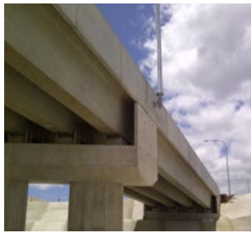
Prestressed decks and girders 53
