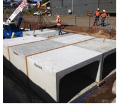
Box culverts - small 16
