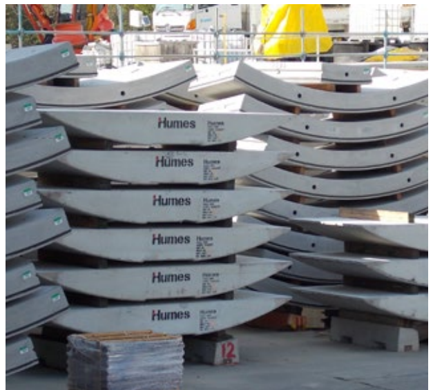
Tunnel invert units
