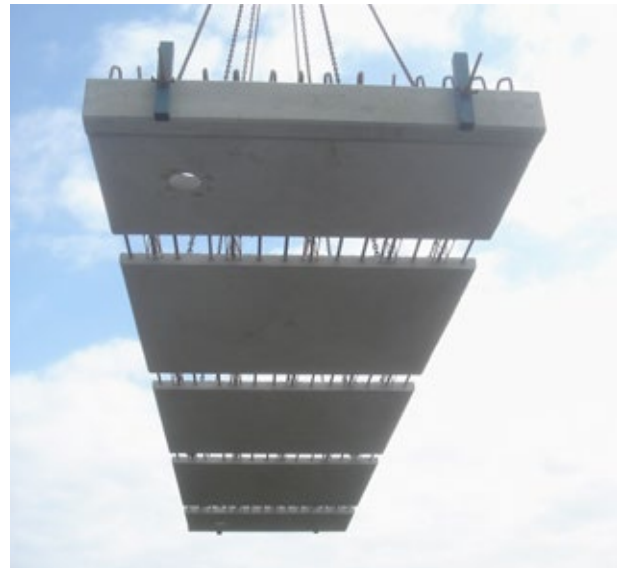
HumeSlab® bridge deck unit
