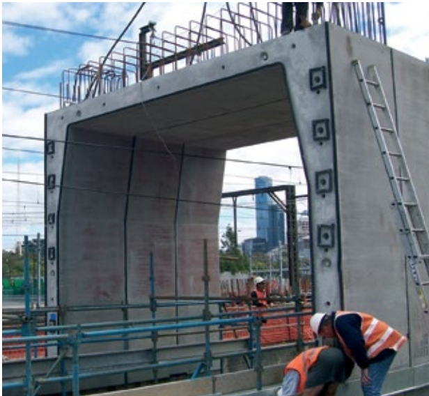
Box culverts with post-tensioning ducts
