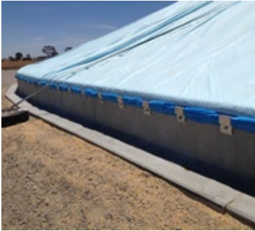
Grain bunker modules
